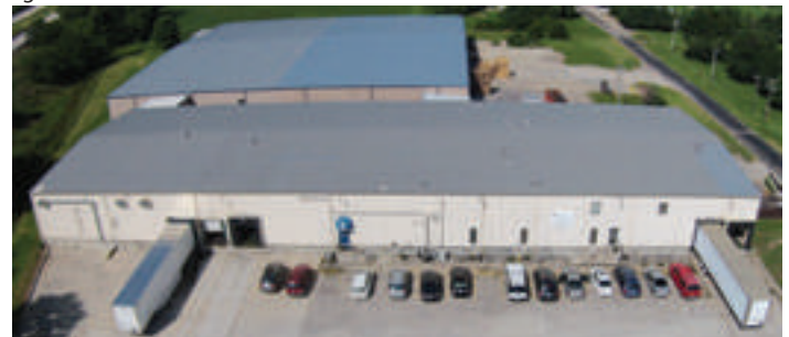
BK Resources' 75,000 sq. ft. Headquarters, Warehouse & Distribution Center, Altamont, IL
